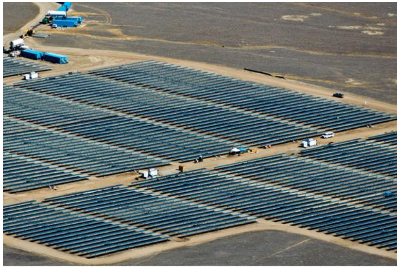
California Valley Solar Ranch, photo by SunPower
