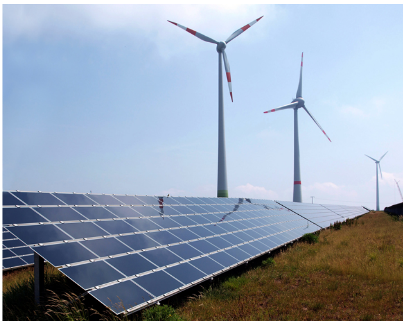
Wind and solar in Germany, photo by Kubelbeck
